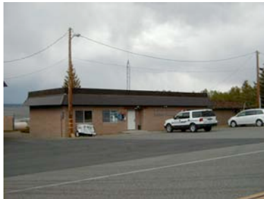
Sheriff's Crowley Lake Substation.
