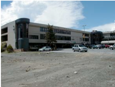
In Mammoth Lakes, the Probation Department is located in the Sierra Center on the 3 rd Floor.
