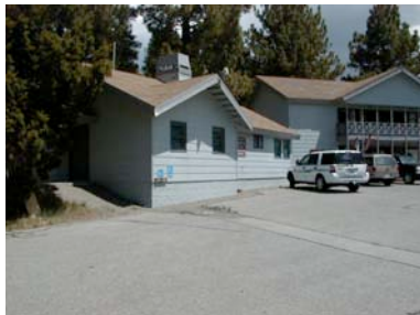
Sheriff's June Lake Substation.
