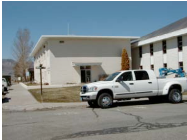
The County Administrator's Office is located on the 1 st Floor of Annex I in Bridgeport.
