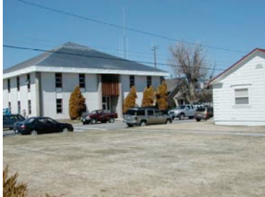
Information Technology is located on the 2 nd Floor in Annex II in Bridgeport.
