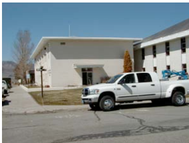
Public Works Administration is located on the 2 nd Floor of Annex I in Bridgeport.
