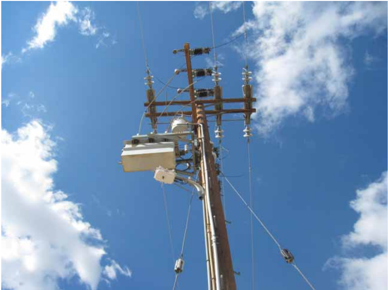
Power pole on west side of Highway 6 located mid parcel.
