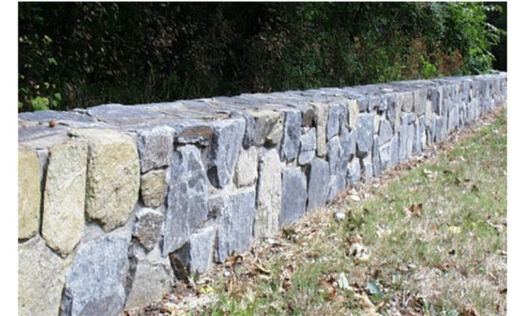
A Stone Masonry Guardwall consists of concrete faced with natural stone. Above: Caltrans guardwall in San Luis Obispo.
