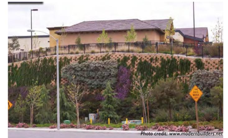
The VERDURA Living Retaining Wall system is a fully plantable block wall that is Caltrans approved. Photo credit: www.modernbuilders.net
