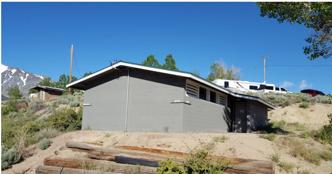
Figure 41. Public restroom, view toward southwest.
