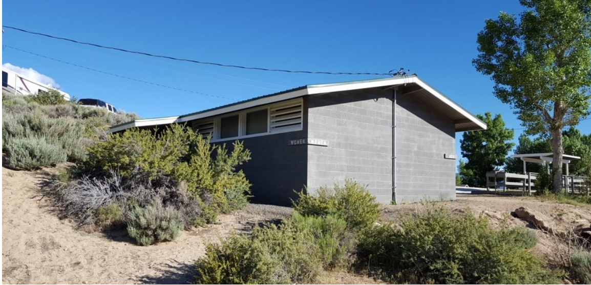
Figure 40. Public restroom, view toward northwest.
