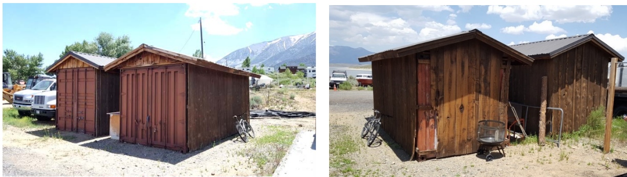
Figure 31. Metal shipping containers within old-wood shelters. Left: front, view toward southeast. Right, back, view toward northeast. Note how tightly the covering sheds fit the containers.
