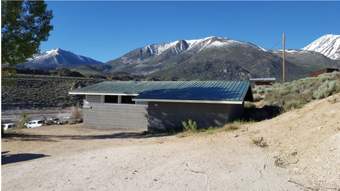
Figure 42. Public restroom, view toward south.
