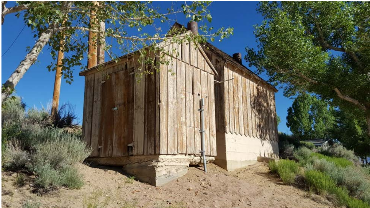
Figure 46, below. Smaller LADWP building center left, view toward northwest. Larger LADWP to right.
