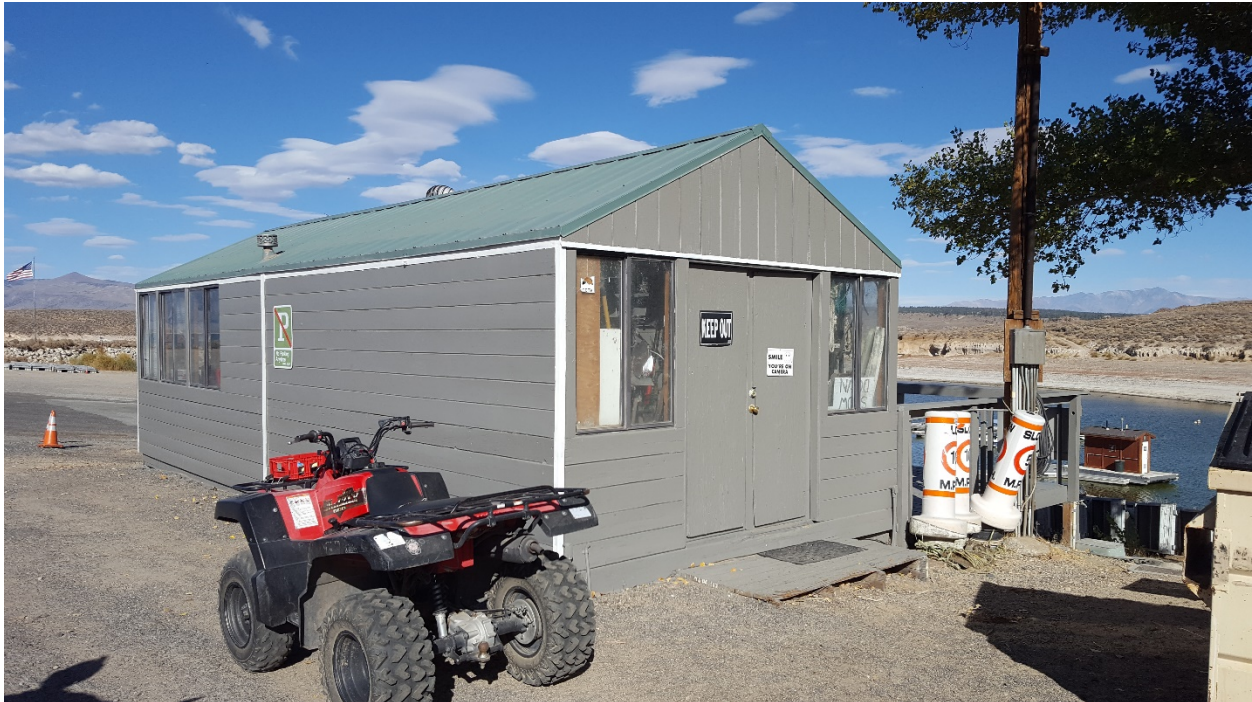
Figure 39. Boathouse/Storage Building, view toward northeast.
