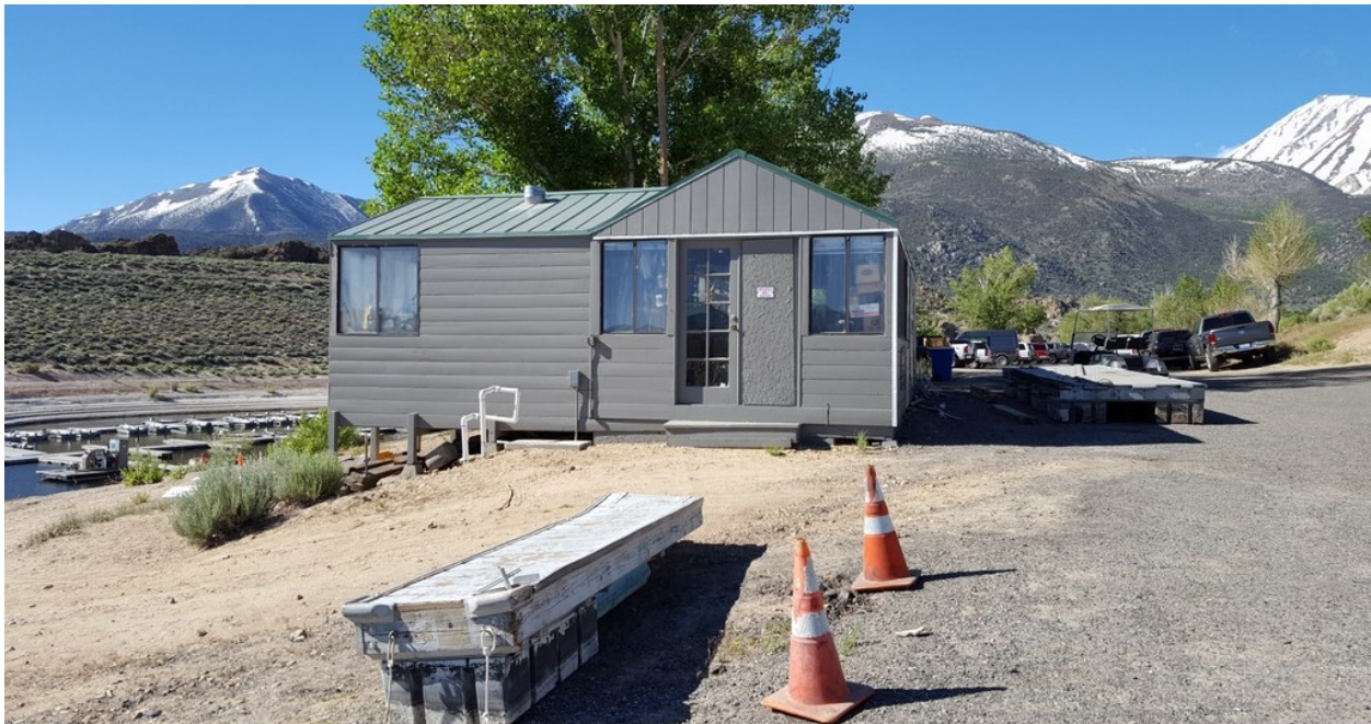
Figure 37. Boathouse/Storage Building, view toward south.
