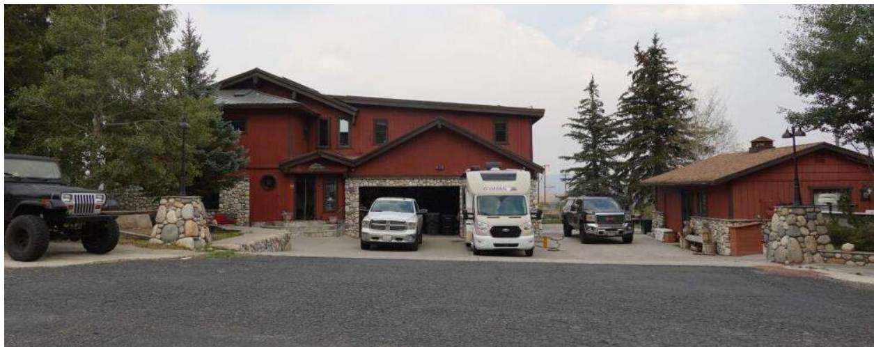
Figure 5: Street View of 90 Aspen Place
