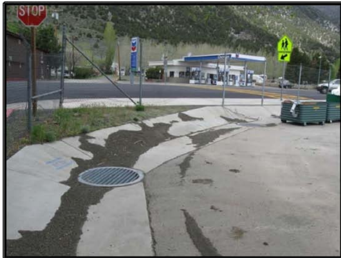
#4 – Caltrans yard drainage improvements
