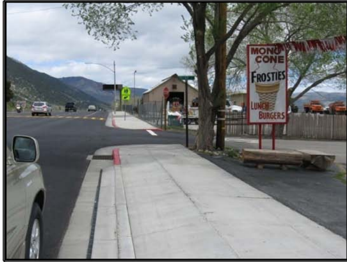
#3 – Stormdrain with slotted drain in foreground
