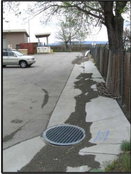
#4 – Caltrans yard drainage improvements. Sand trap located in background.
