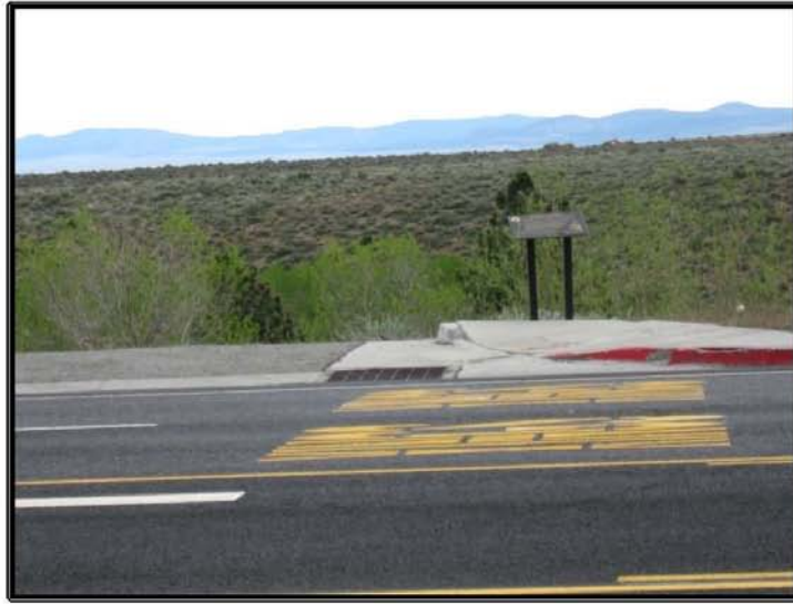
#13 – Stormdrain near Rush Creek. Exits to underground infiltration via perforated pipe.
